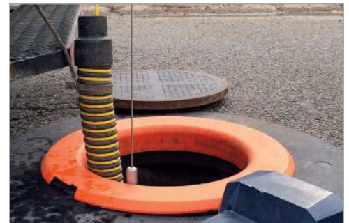
Sewer jet hose and camera protection
